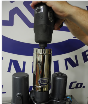
2. Place Impact Wrench Into Socket & Remove Cap
